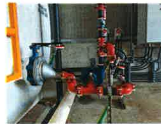
Figure 6 –New Installation Piping
