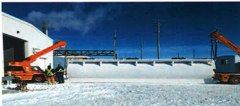
Figure 4 – Install of new 10,000 USG Horizontal Tank with Agitators.
